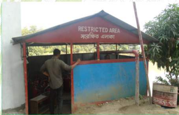
Water pump for fire control
