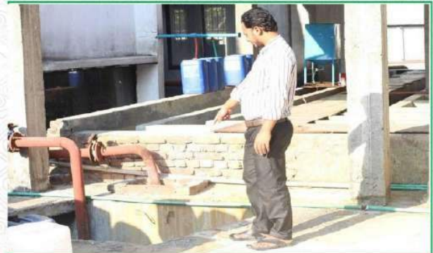
4) An aerobic Digester 1
